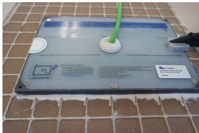
Figure 5: Spreading the mounting adhesive
